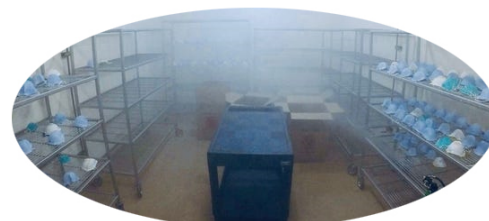
Fogging PPE Equipment
